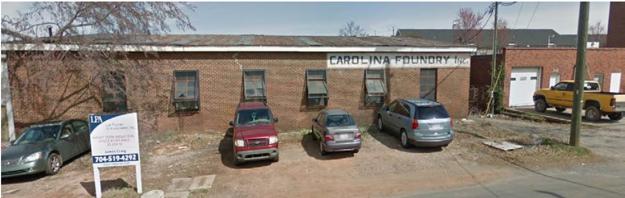
The subject property is developed with a warehouse use.
