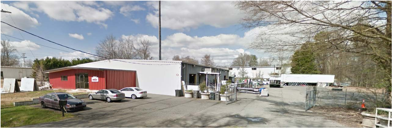
The subject property is developed with a warehouse use.
