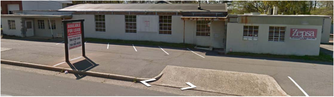
The subject property is developed as a warehouse.
