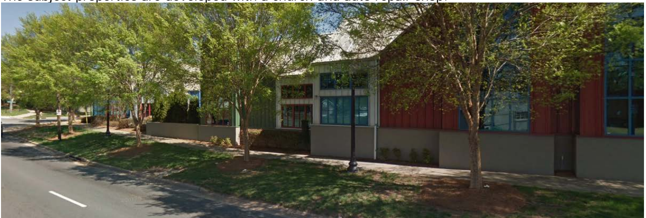
The property across South Tryon Street is developed with office uses.
