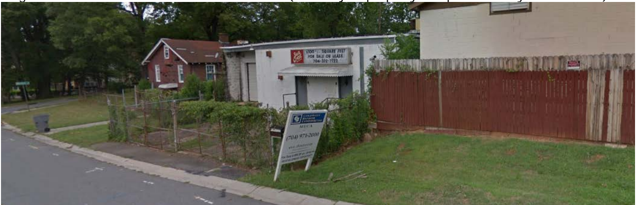
Properties to the north across Worthington Avenue are developed with warehouse uses and single family. The single family homes are located within the Wilmore Historic District.
