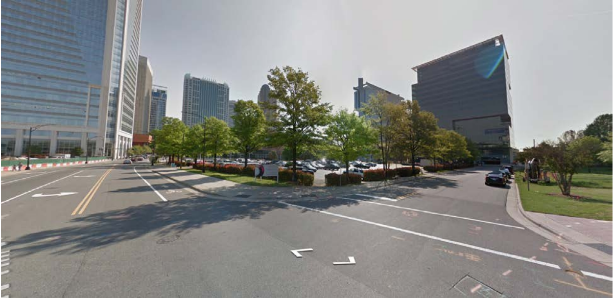
The commercial structures on the site are currently being demolished (view from East Hill Street and South Tryon Street).
