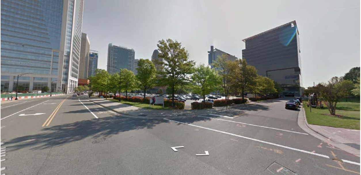
The commercial structures on the site are currently being demolished (view from East Hill Street and South Tryon Street).
