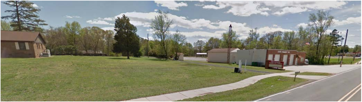
The adjoining properties along Mount Holly-Huntersville Road include a single family home and a volunteer fire department.
