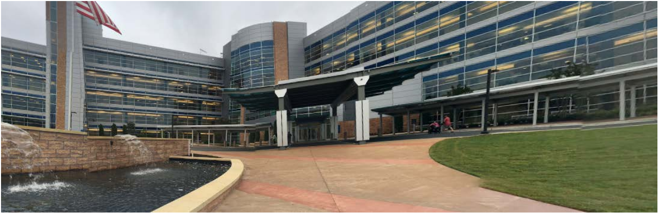
The Charlotte Veterans Health Care Center is located to the north and east of the site.
