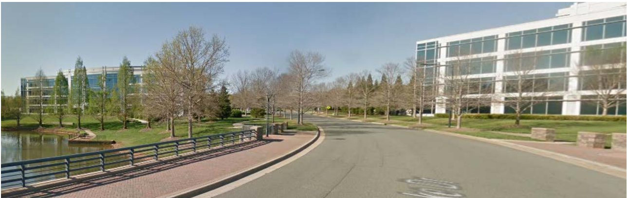
The Lake Pointe office park is located to the west.
