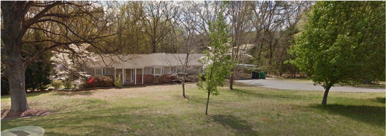
The subject property is developed with single family homes and the remainder of the tract is vacant.
