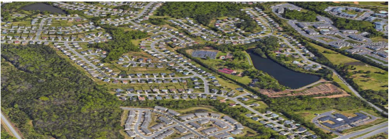
Properties to the northeast across South Tryon Street are developed with multi-family and single family homes.
