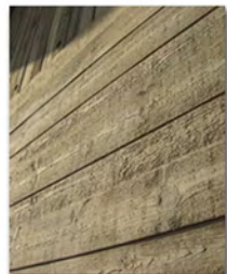
BOARD FORMED CONCRETE
