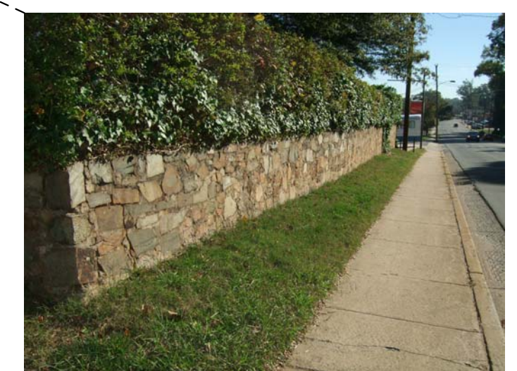
EXISTING RETAINING WALL AND SIDEWALK
