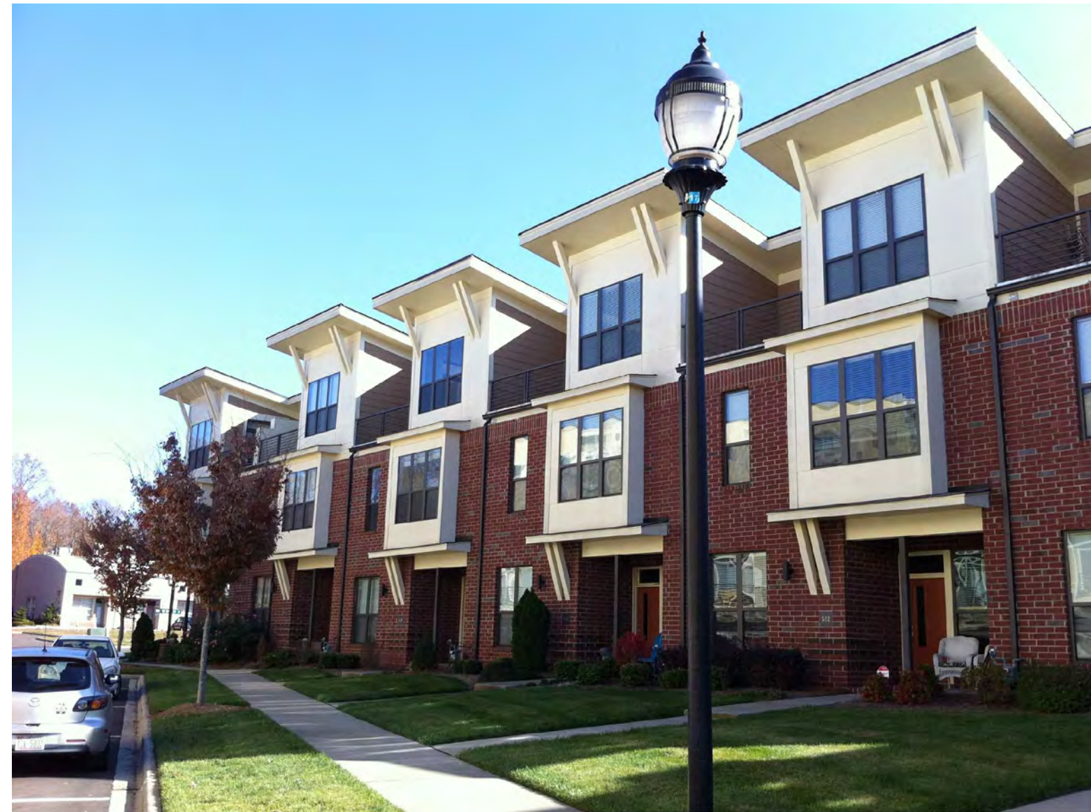
INTERNAL STREET — MAIN VIEW — BUILDING TYPES 'A' & 'B' FRONT NOT TO SCALE
