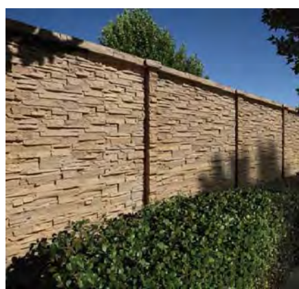
Precast Concrete Wall with Stone Finish* *Stone finish, style and quarried stone caps to be agreed upon with the abutting neighbor.
