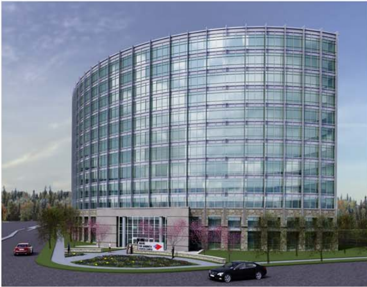
NORTH TRYON & WEST MALLARD CREEK CHURCH ROAD INTERSECTION
