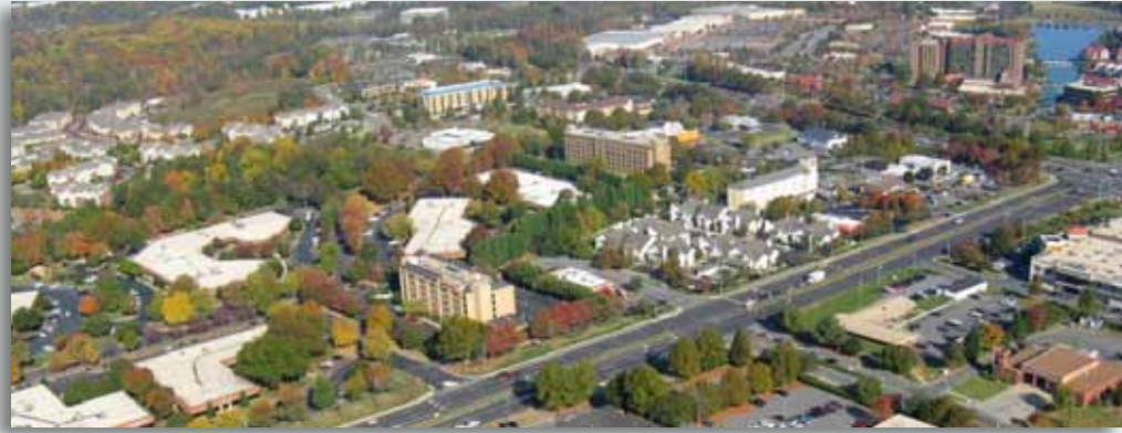
North Tryon Street's existing wide median will be the location of the LYNX Blue Line Extension rail line.
