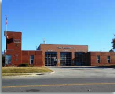
Fire Station 27 protects UNCC, hotels, retail centers, and community residences.
