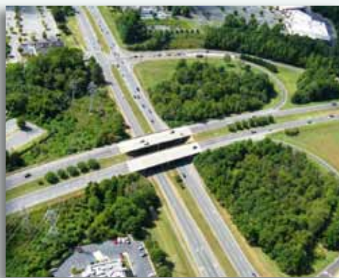
Two major thoroughfares intersect - W.T. Harris Bv crosses over University City Bv.
