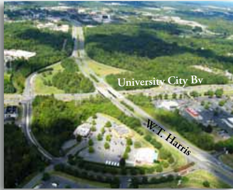
Retail and Phase 2 Toby Creek Greenway converge at W.T. Harris and University City boulevards.
