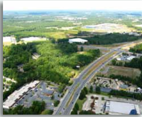
Road improvements, including the "Weave", benefits existing and future land uses.
