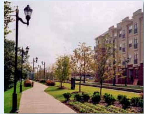
A pedestrian pathway, with landscaping and lighting, runs alongside the South LRT line.
