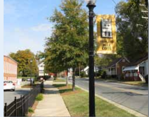
Highland Mill (1904) textile mill, has already converted to apartments and retail space.
