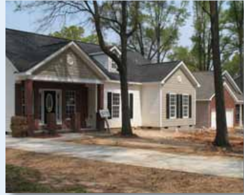
New construction on Neal Drive near the Tom Hunter station site.
