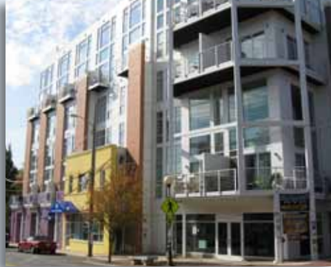
New development in the arts district is located across the street from 1927 store fronts.
