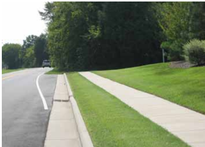
Sidewalks are being built along parts of Sledge Road by developers of adjacent property. A “farm-to-market road upgrade” may complete remaining gaps as part of a future City capital project.
