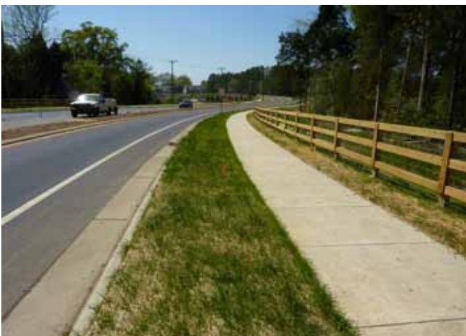
Shopton Road West near Steele Creek Road is an example of a newly improved thoroughfare, including new turn lanes, median islands, bicycle lanes, planting strips and sidewalks.
