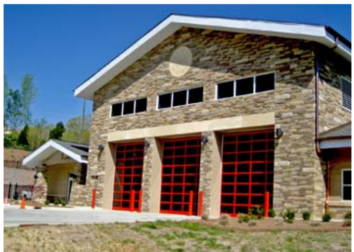
Station 38 on Shopton Road West serves the growing residential and industrial development in the Westinghouse Blvd area.
