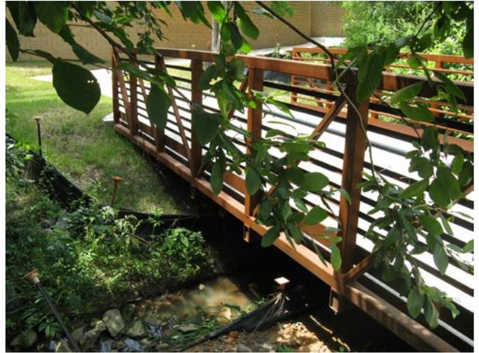
**6A** A bridge is used to connect across the creek, rather than a culvert.
