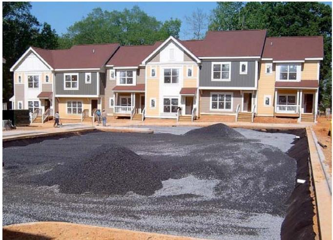
**3G** Construction of a pervious parking area to serve these townhomes will minimize stormwater runoff, providing a “green” alternative to traditional pavement.
