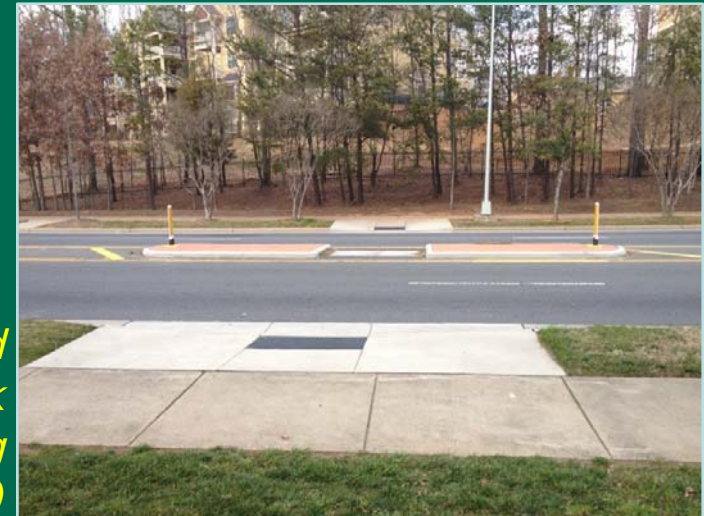
Tyvola Road Mid-Block Crossing (Completed)
