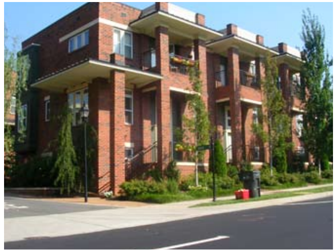
This newer multi-family development is compatible in scale and massing with surrounding buildings on Hawthorne Lane.
