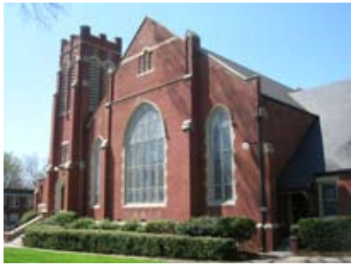
5 Hawthorne Lane United Methodist Church
