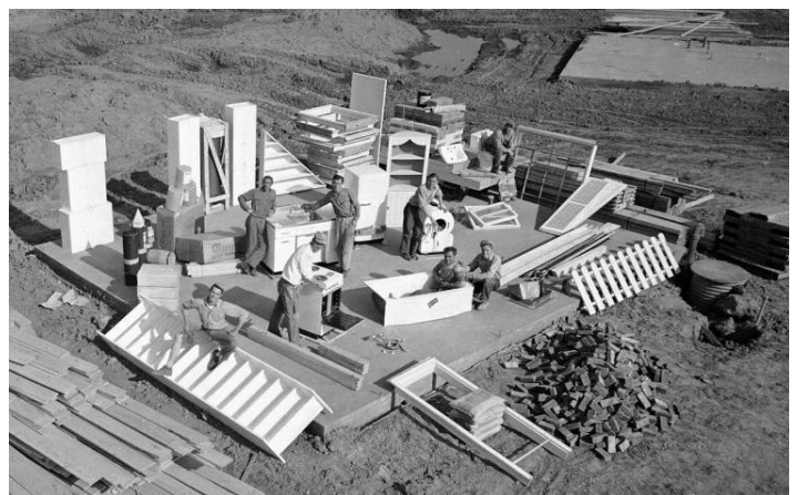
Above: Levittown, NY is one of many suburban developments built after WWII for returning veterans and their families. Home production was modeled in an assembly line manner and thousands of identical homes were produced easily and quickly.
