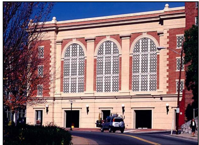
Facade Treatment on Parking Deck
