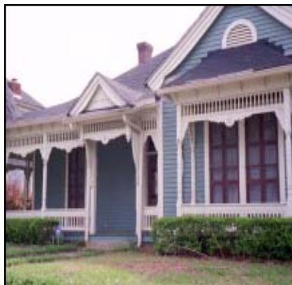
The use of brackets, gable vents or other architectural details is strongly encouraged.
