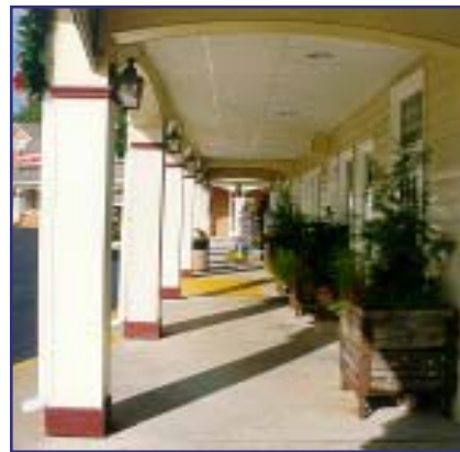
Canopies and awnings may extend over the public sidewalk provided obstructions are kept to a minimum clear height of 8'.
