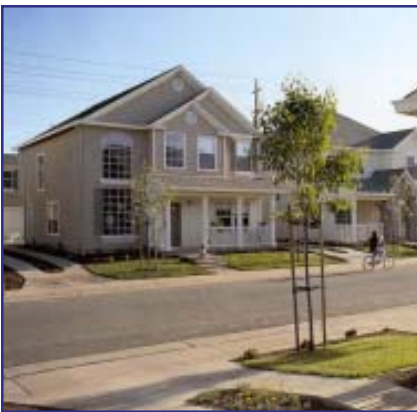
Front Doors should be visible from the street.
