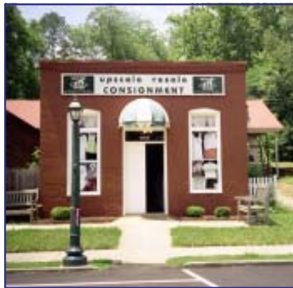
Building facades should be articulated with canopies, porches, cornices, roof lines and window details to avoid monotonous blank facades.
