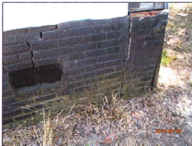
1.1 Item 1(Picture) RIGHT REAR CORNER
