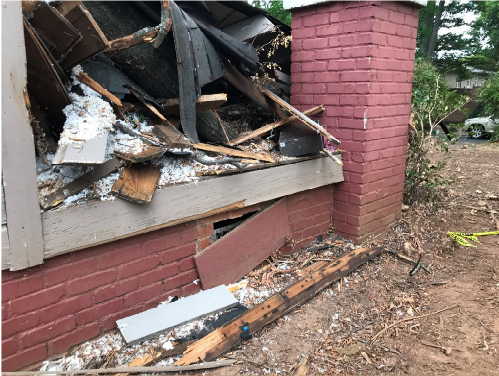
Photograph 11: Two front brick columns are leaning.
