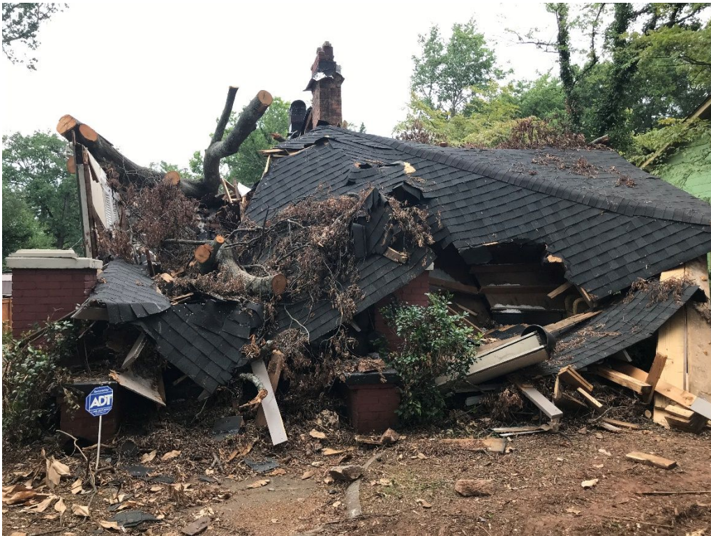
Photograph 4: The current east (front) elevation with the collapsed roof and walls.
