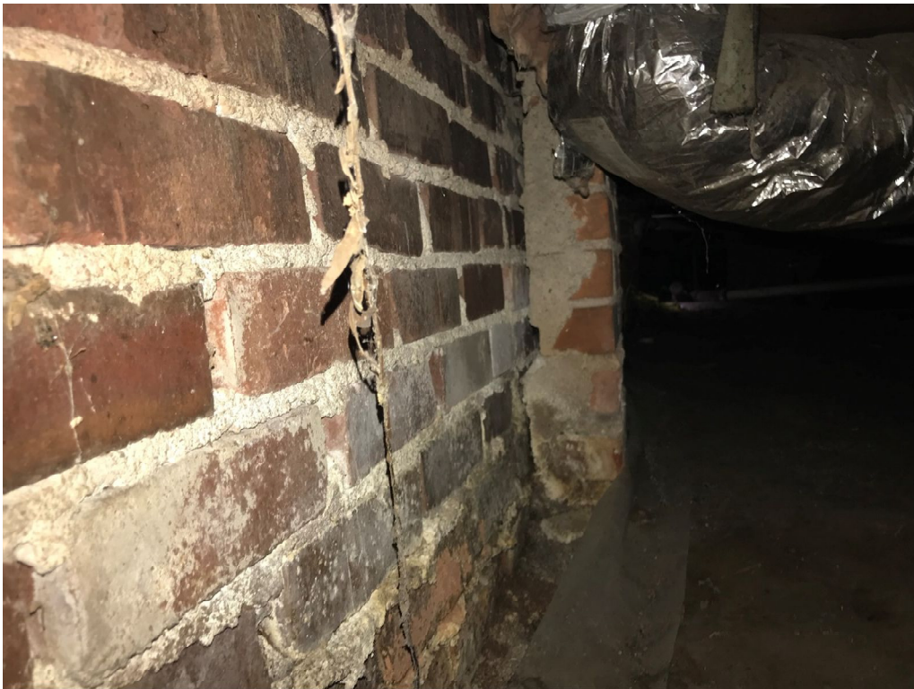
Photograph 10: Single wythe curtain wall with single brick thickness pier.
