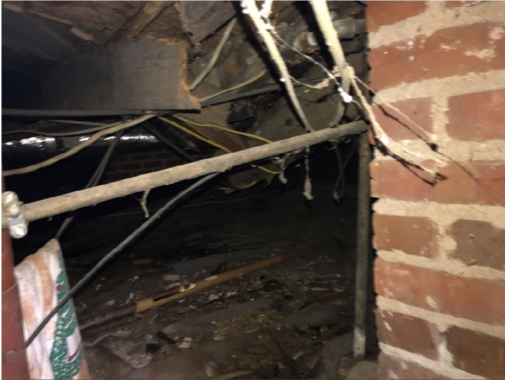
Photograph 9: Additional cracked floor joists.
