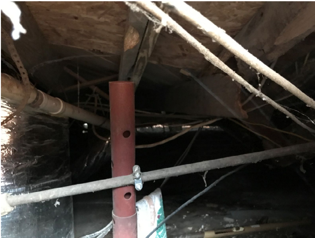
Photograph 8: Displaced and cracked flooring and supplemental piers.
