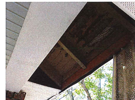
exposed rafters beneath vinyl
