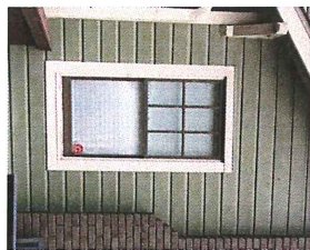
EXISTING WINDOW/TRIM/SIDING DETAIL: MATCH NEW WINDOWS W/ EXISTING MATERIALS AND DETAILS, VIF
