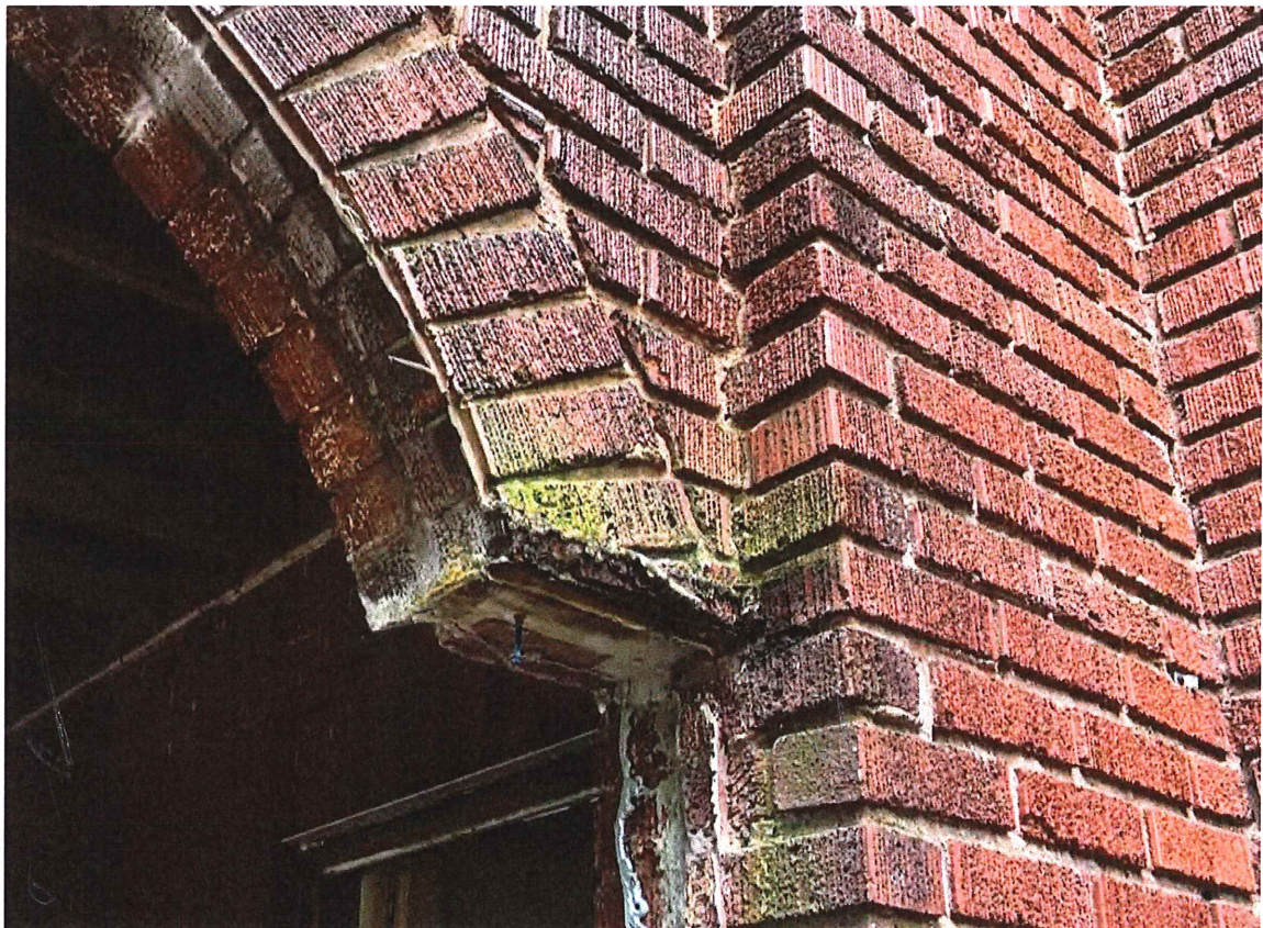
Photo Showing Solid 2-Wythe Brick Wall After Existing Door Was Removed
