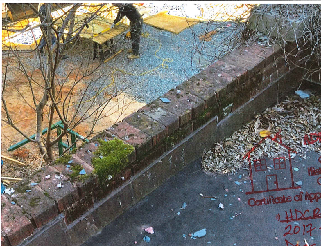
Photo Showing Top of Wall Where Limestone Coping is Missing at Rear of Brick Parapet
