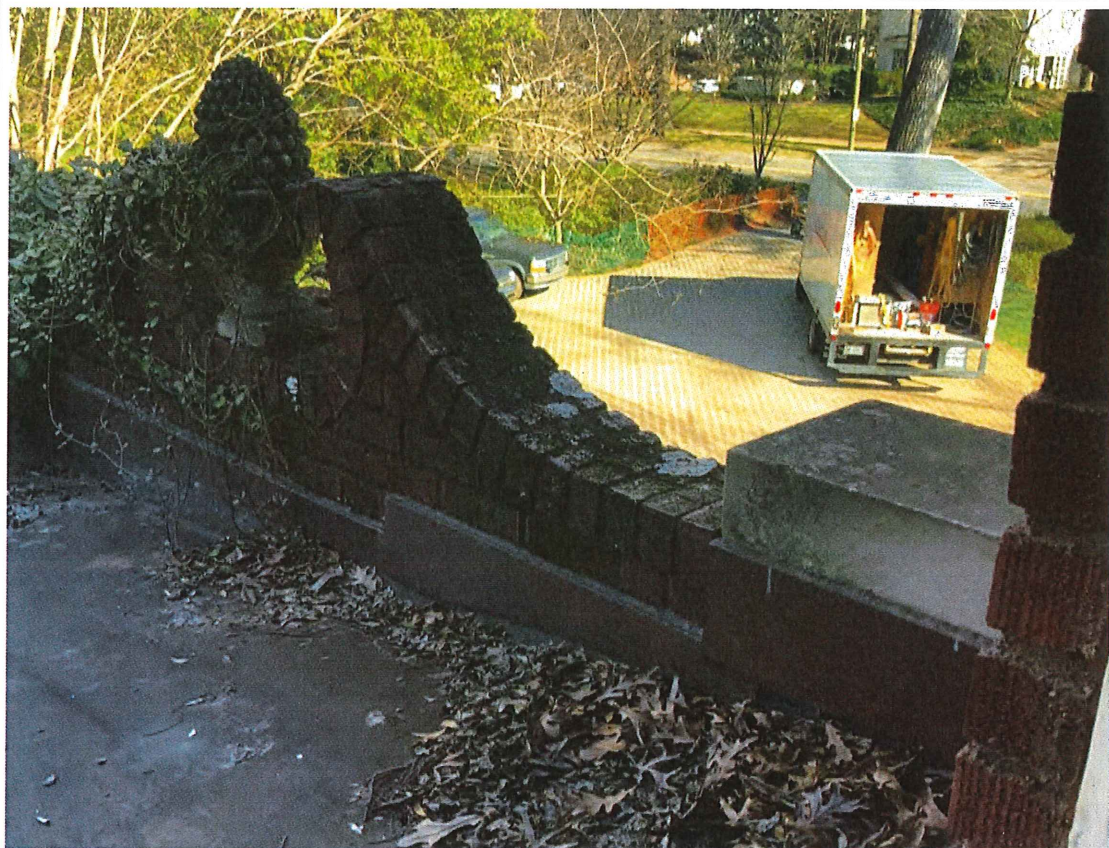
Photo Showing Existing Flashing at Back of Brick Feature
