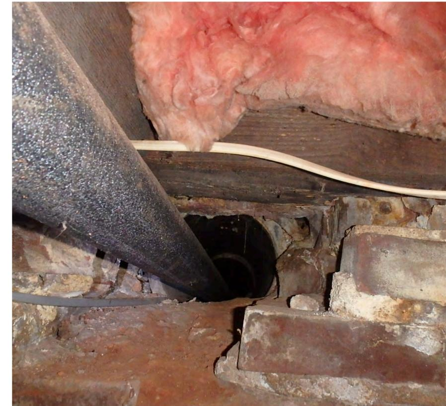
Wood Band (Behind Ledger) is Severely Decayed
