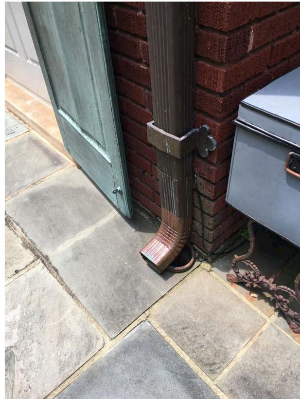
Downspouts Bypass Integrated Drains, Indicating Previous Drainage Problems
