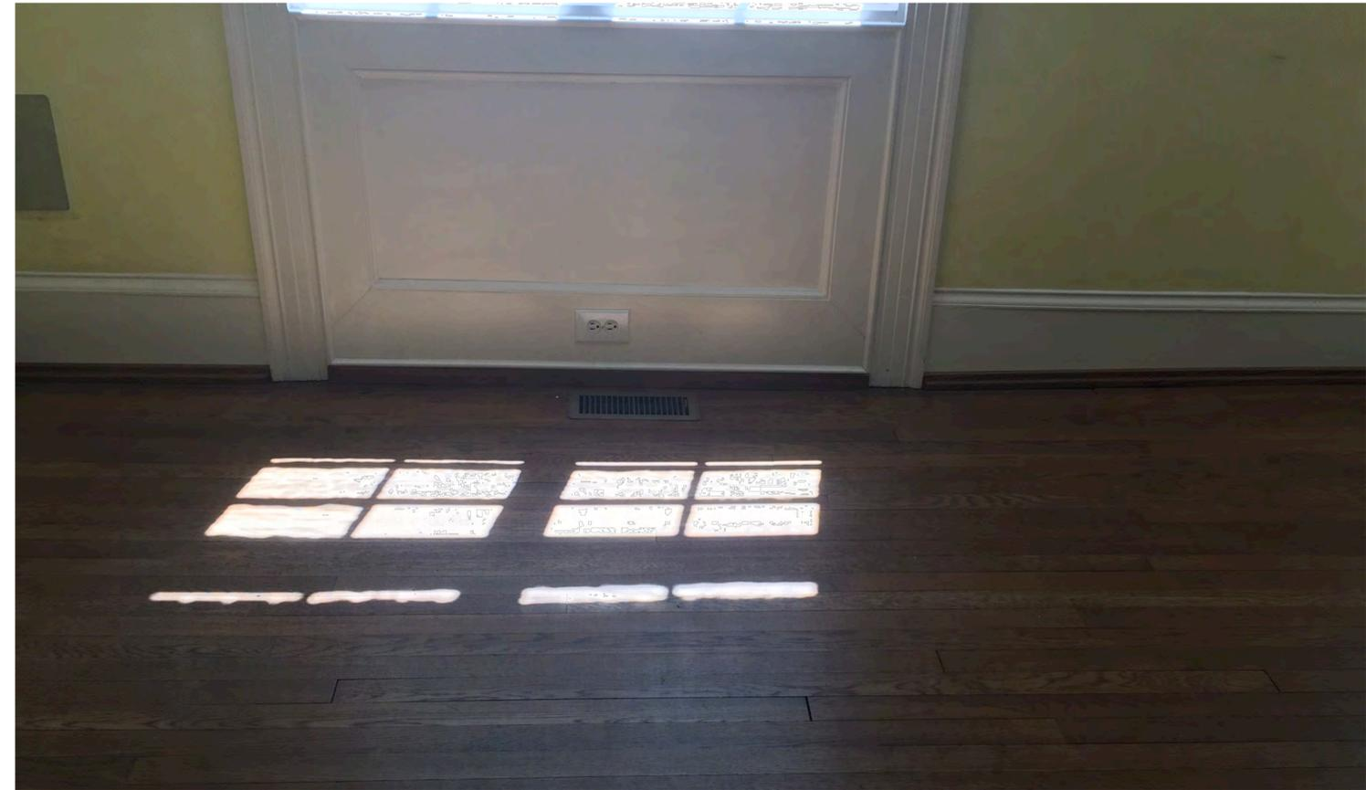
Point Loads Next to Windows are Sinking into the Floor, Indicating Structural Damage Below
