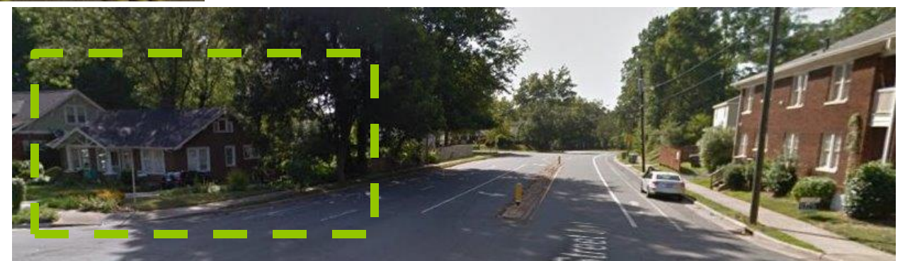
APPROACHING 404 WALNUT FROM W. 4 TH ST.
