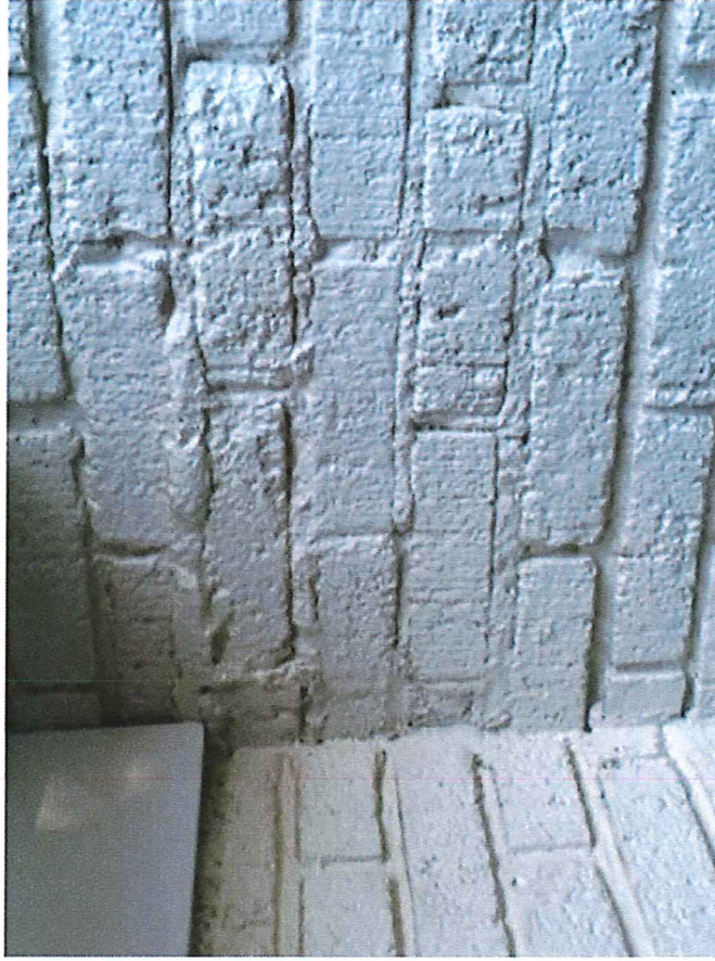
Despite being painted, this mismatched butt joint on the SW side, between the original house (right) and the 2006 addition (left), is clearly evident. Note once again the uneven rows of brick at the joint. The abundance of unsightly-and potentially damaging-mortar overfill on the upper right wall speaks for itself.
