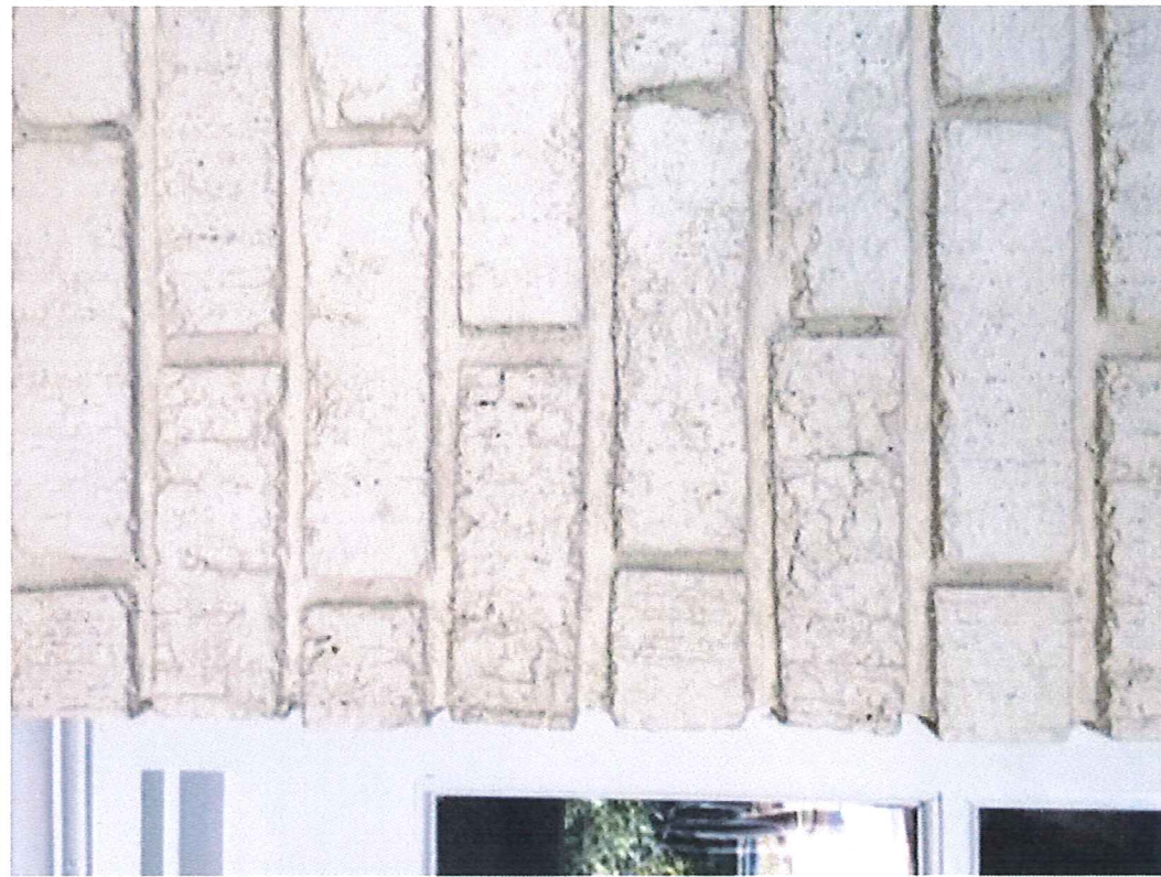
Uneven head & bed mortar joints, crooked & broken bricks- right wall of 2006 rear addition
