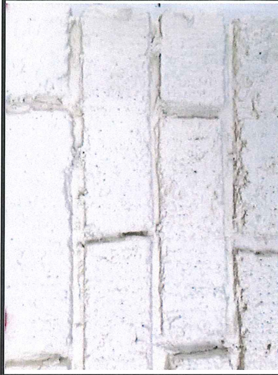
Top of crooked NW wall soldier course, protruding 1/4" - 1/2" from rest of wall-exposing it to standing water.
