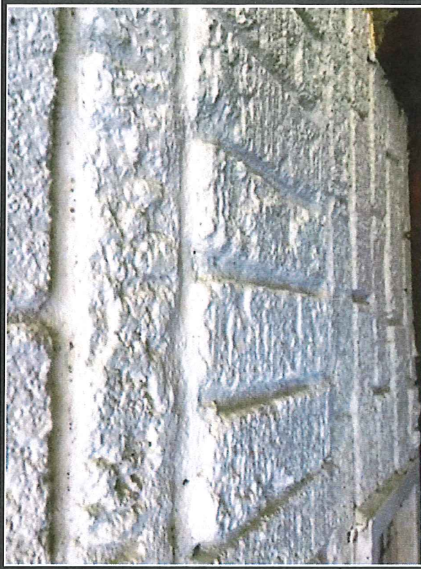
Top of crooked NW wall soldier course, protruding 1/4" - 1/2" from rest of wall-exposing it to standing water.
