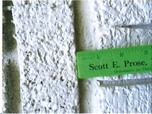
SW wall of 2006 rear addition. One of many head & bed mortar joints one inch wide. (industry standard is 3/8")
