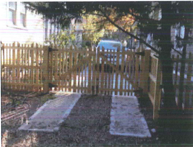
Rear yard fence and gate facing street
