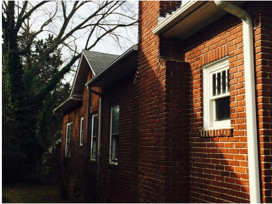
Left Side of house-no changes to windows.
