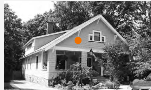
Wood is used extensively for siding and trim (top), trim on masonry buildings (center) and shingle siding (bottom). The wide variety of size and detail is dependant on the style of the building.
