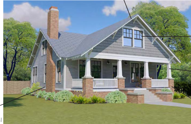
Cross gable roof with deep eaves and brackets
