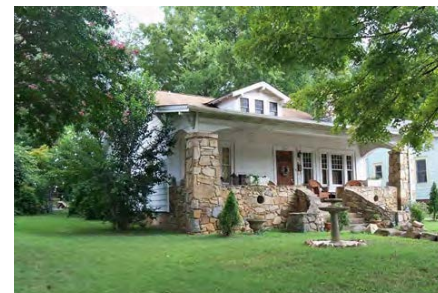
This traditional bungalow has a side gable roof with a shallower pitched section covering the front porch.
